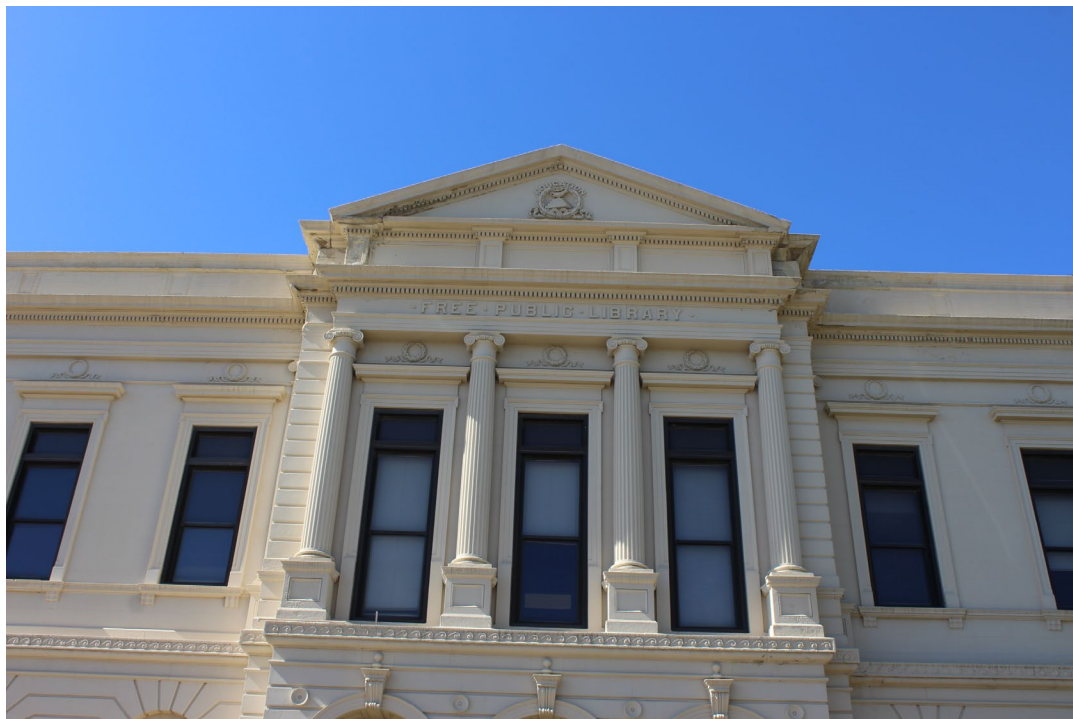
Existing signage on the south elevation.
